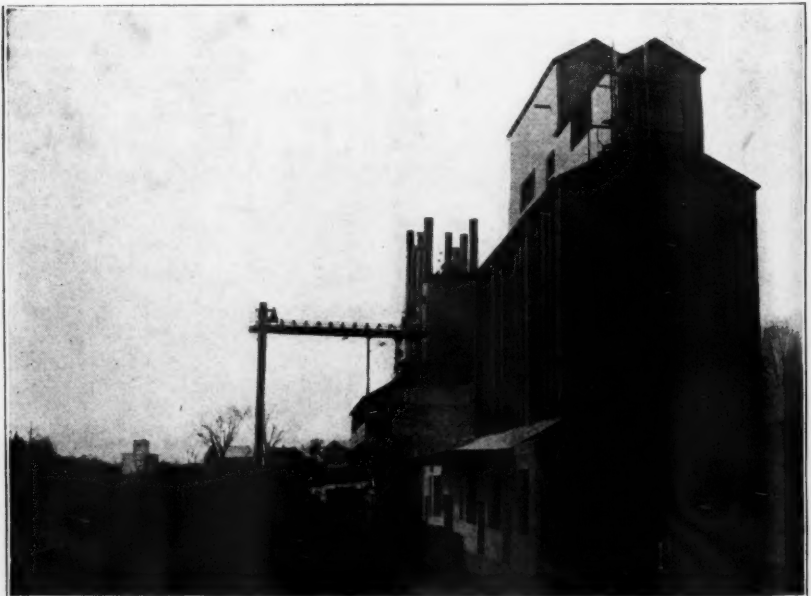
The Storage and Packing Plant.
